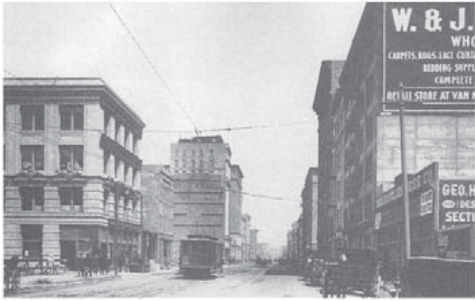
Fig. 1. A 1908 photo of the newly rebuilt Mission Street in the vicinity of Yerba Buena Gardens. (California Historical Society, San Francisco, in Bloomfield, p. 385)
